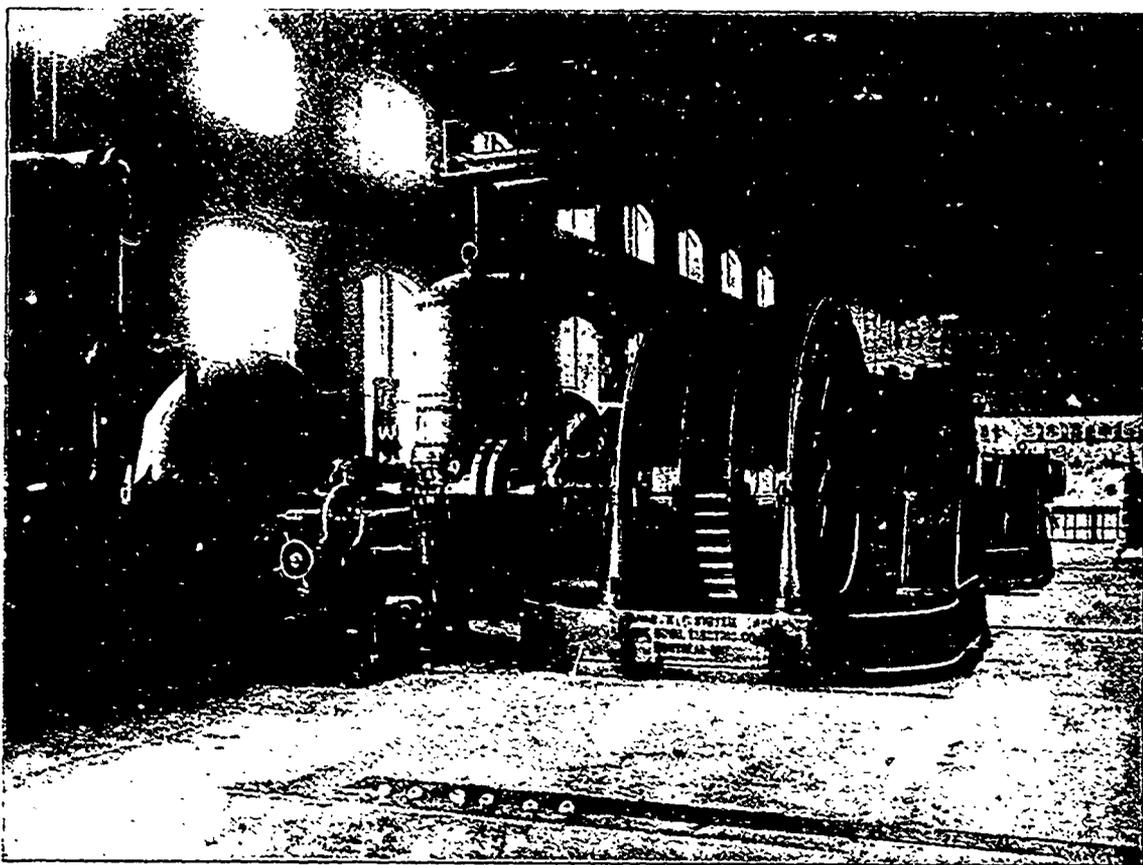
1000 K.W. "S.K.C." DIRECT CONNECTED UNITS—CATARACT POWER COMPANY'S PLANT.
