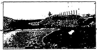
FIG. 1. ARRANGEMENT OF HEAD GATES.
