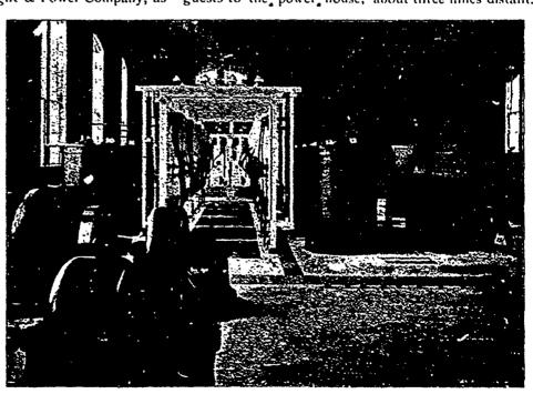
FIG. S. HIGH VOLTAGE SWITCHBOARD, STEP-UP TRANSFORMERS AND EXCITERS.
