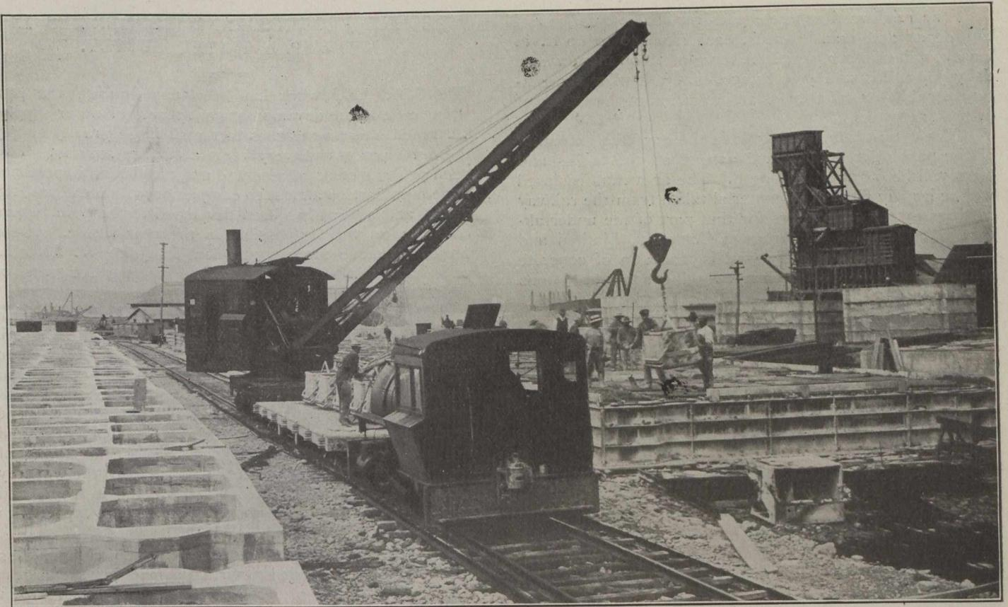
Fig. 6.—Filling the Forms with Concrete.
