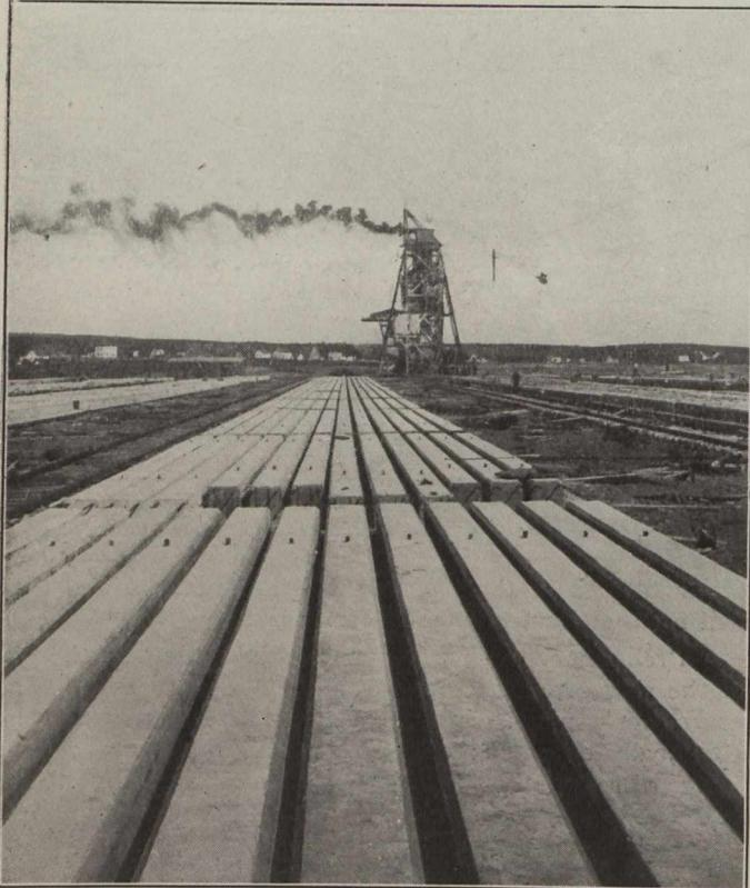
Fig. 7.—Making Reinforced Concrete Piles.
