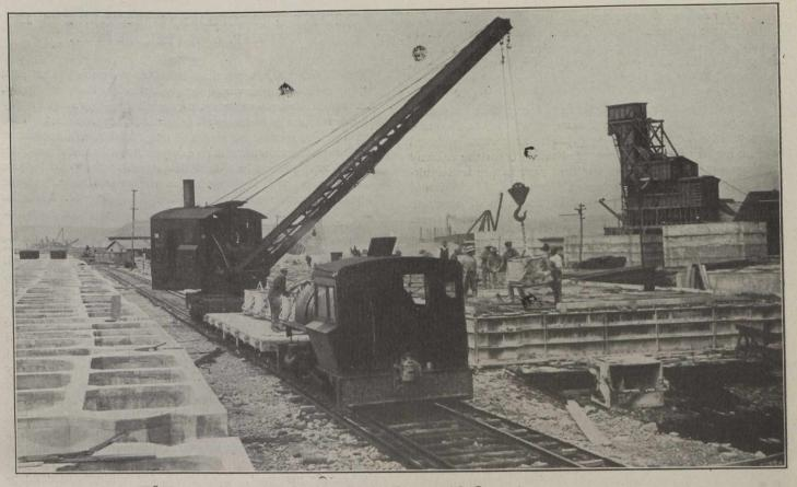
Fig. 6.—Filling the Forms with Concrete.
