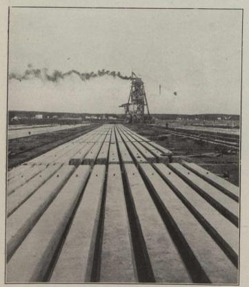
Fig. 7.-Making Reinforced Concrete Piles.
