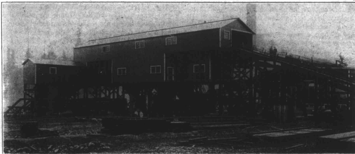
The Tipple at Granby's New Coal Mine, Cassidy, Vancouver Island.
