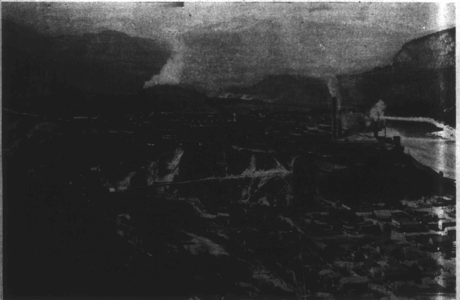
General View, Consolidated M. & S. Co. Smelter, Trail, B.C.
