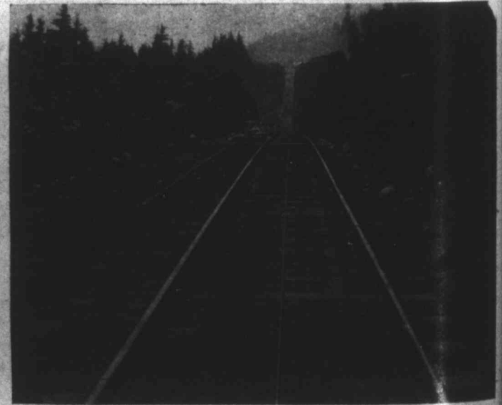
Incline to Mill—Note 1½ inch wire cable used to haul skips. Incline is 1,500 ft. from top of mill and is 5,400 ft. long.
