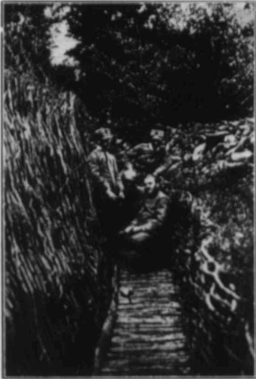
Italian branches elaborately constructed with lattice work of branches to keep the earthwork from caving in. The Italians are pressing forward onto the Austrian outpost of Trieste.
