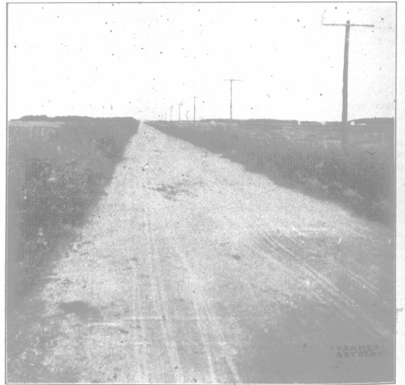
GOOD ROADS IN STONEWALL DISTRICT.
