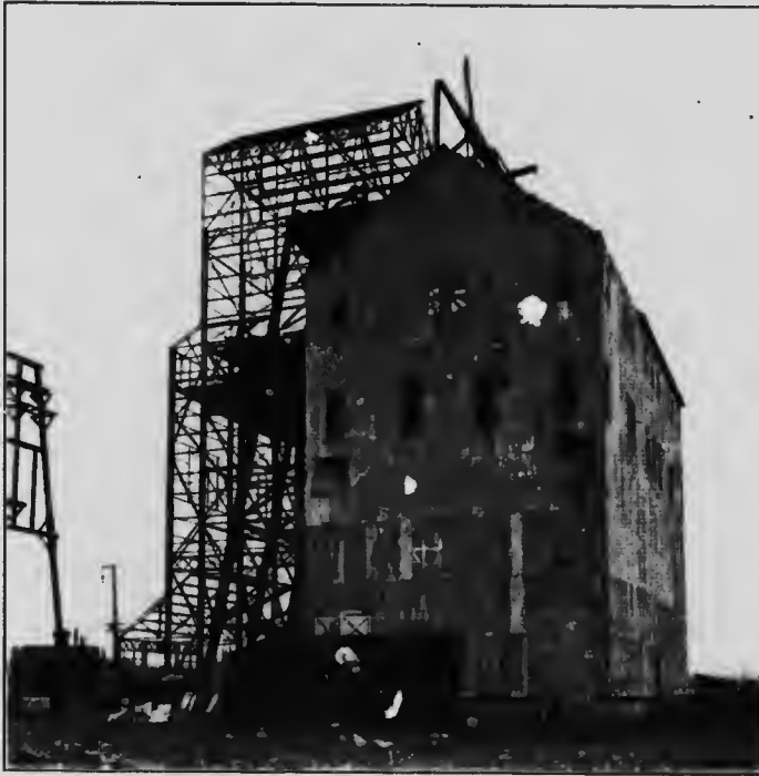
HEAD-FRAME. TAMARACK, No. 2. SHAFT.
