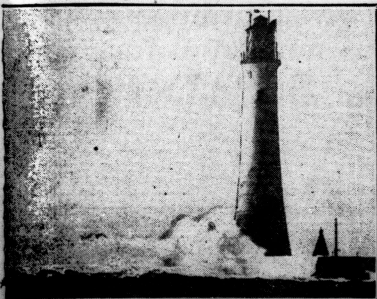
On Wolf Rock is said to be the world's most dangerously situated lighthouse in the world. Without a moment's warning, a huge sea, sufficient to wash away three tons of supplies, as once happened, will sweep across the landing
