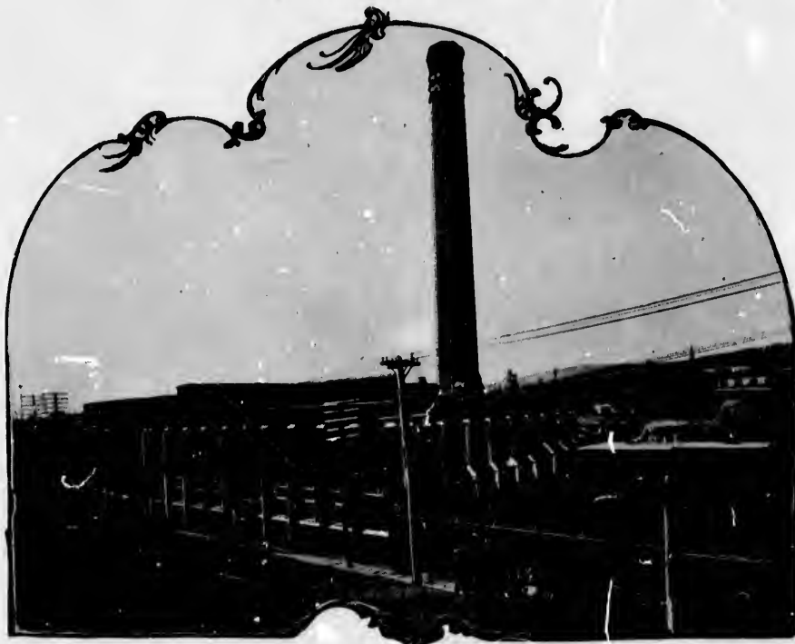
POWER HOUSE, MONTREAL STREET RAILWAY.
