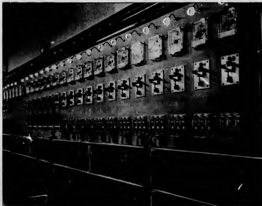
SWITCH BOARD, POWER HOUSE, MONTREAL STREET RAILWAY.
