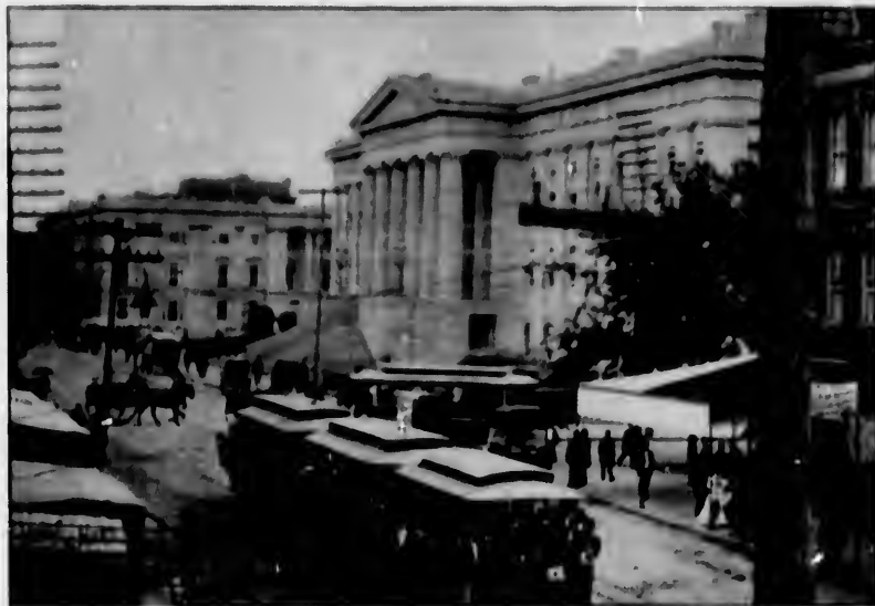
LOADED FOR HOUSE HALL—SEVENTH STREET CABLE RAILWAY, WASHINGTON, D.C.
