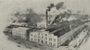
NEW FACTORY BUILT IN 1895 SINCE THEN THE FOLLOWING EXTENSIONS HAVE BEEN MADE MACHINE SHOP LENGTHENED 140 FT. NOW 448 x 123 BOILER SHOP 100 FT. NOW 230 x 80 WITH CORRESPONDING INCREASE MOULDING SHOP 100 FT. NOW 180 x 80 INCREASE BLACK SMITH SHOP 40 FT. NOW 180 x 48 IN EQUIPMENT.
