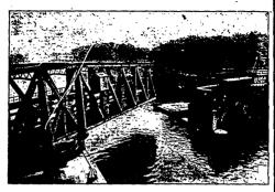
AQUEDUCT BEING SWUNG ASIDE TO ALLOW VESSEL TO PASS ON SHIP CANAL BENEAT seen in the first illustration on this page
