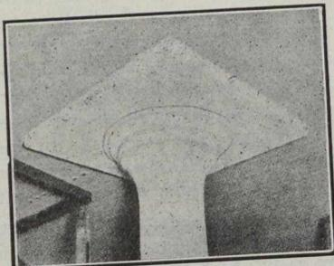
Fig. 2.—View of Slab from Below, Showing Column Capital and Several of the Gauge-Points.
