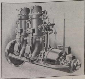
Fig. 5.-Direct Reversible Marine Engine.
