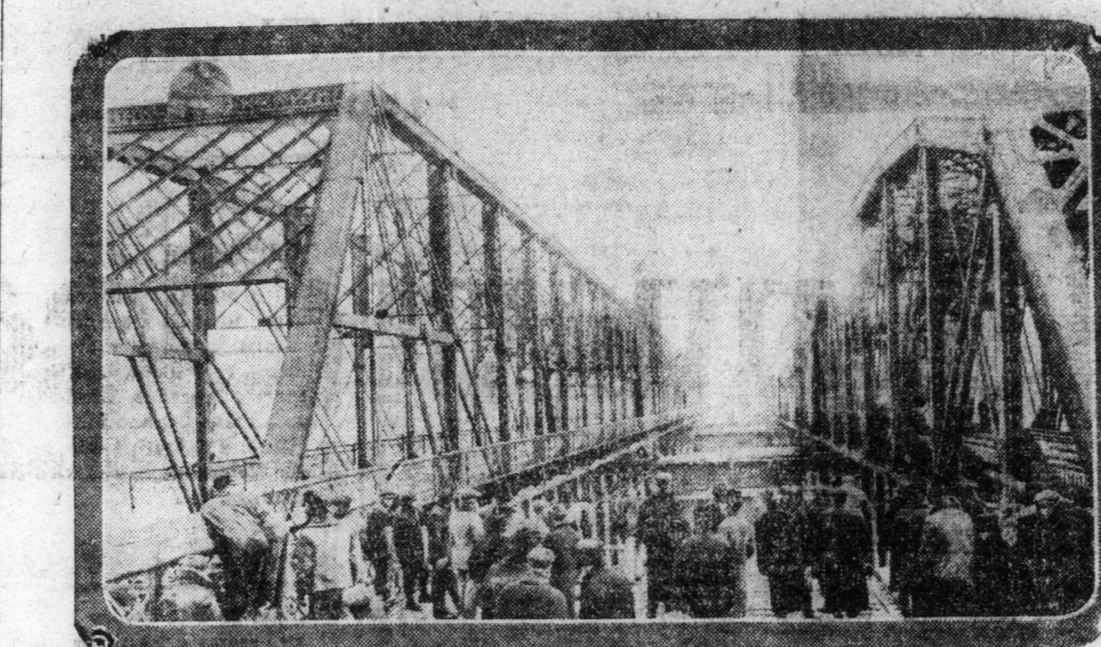
This 11,000,000-pound bridge was moved into position over the Missouri River at Omaha, Nebraska, in exactly 14 minutes, without loss of life or damage to any part of the structure.
