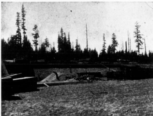
Construction work at the Ladysmith Smelter.
