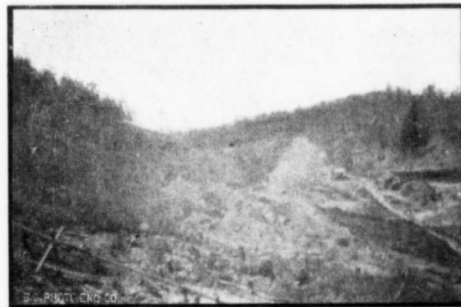
Quarrying at the Snowshoe Mine, Boundary District. The Explosion of a Blast.
