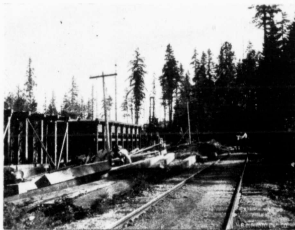
Tyee Ore Bins, Ladysmith, capacity 1,600 tons.
