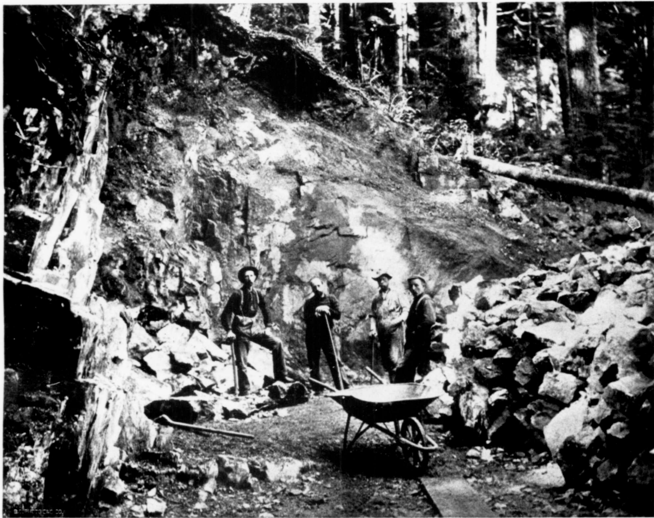
Clyde's Cut, Comstock Mountain—Showing method of quarrying out ore on Yreka property. Part of the dump is seen. All to the left is ore.
