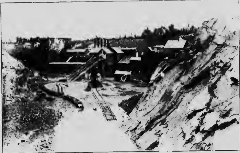
Bathurst mine, Antin Brock, N.S.W.
