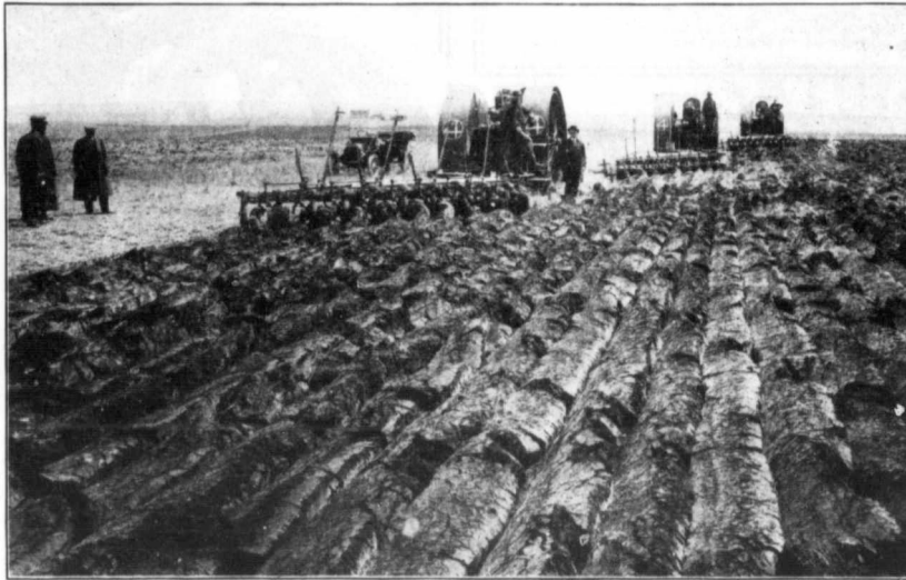
These three Big Four "30s," each pulling ten 14-inch breaker bottoms and turning over 35 feet of furrows at once, broke 8,000 acres of tough prairie sod this summer at the rate of 100 acres a day. The wonderful automatic steering device, an exclusive feature of The Big Four "30," made it possible for one man to run both engine and plows. Write today for "The Book of Gas Traction Engines"—it's mighty interesting.
