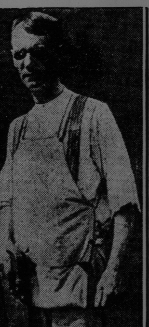
John Taylor of Canton, O., knows how to hit the nail square on the head despite the fact he is blind. He's a carpenter and has just completed a six-room addition to his home. And he did all the work himself. He has built six houses in the 28 years he has been blind.
