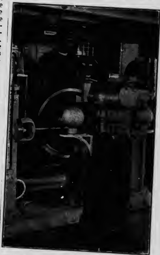
The Wheel on the Bridge Operates the Rudder Several Hundred Feet Away
