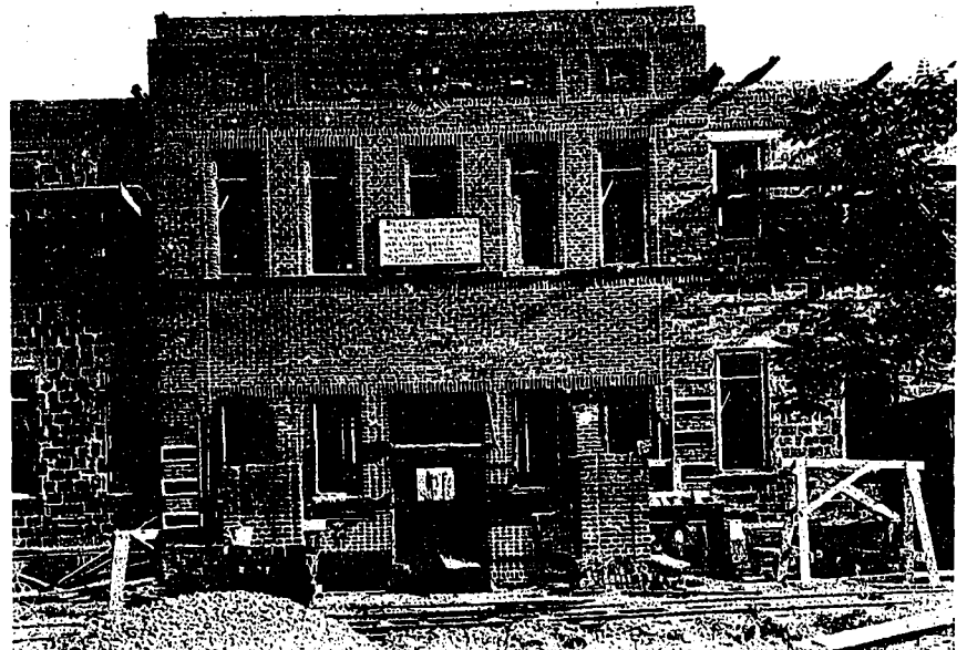
ENTRANCE, INFIRMARY NO. 1, SHOWING USE OF TAPESTRY BRICK AND TILE PATTERNS.
