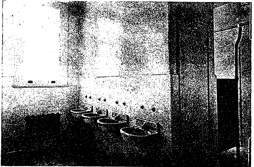
PATIENTS' LAVATORY IN WOMEN'S COTTAGES. NOTE PLUMBING CHAMBER FOR ALL PIPING BETWEEN BASINS AND CLOSETS.
