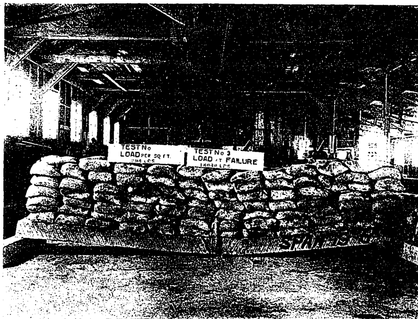
SEIGWART BEAM LOAD TEST. TYPICAL BEAMS FOR ALL DIFFERENT SPANS HAVE BEEN TESTED IN THIS MANNER TO CHECK CALCULATIONS.
