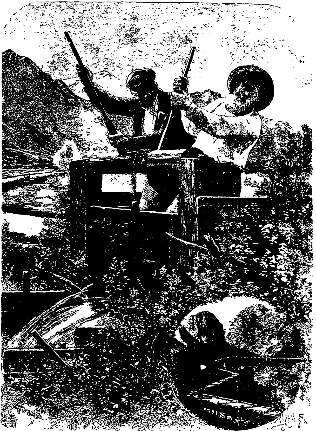
IRRIGATION IN COLORADO.
