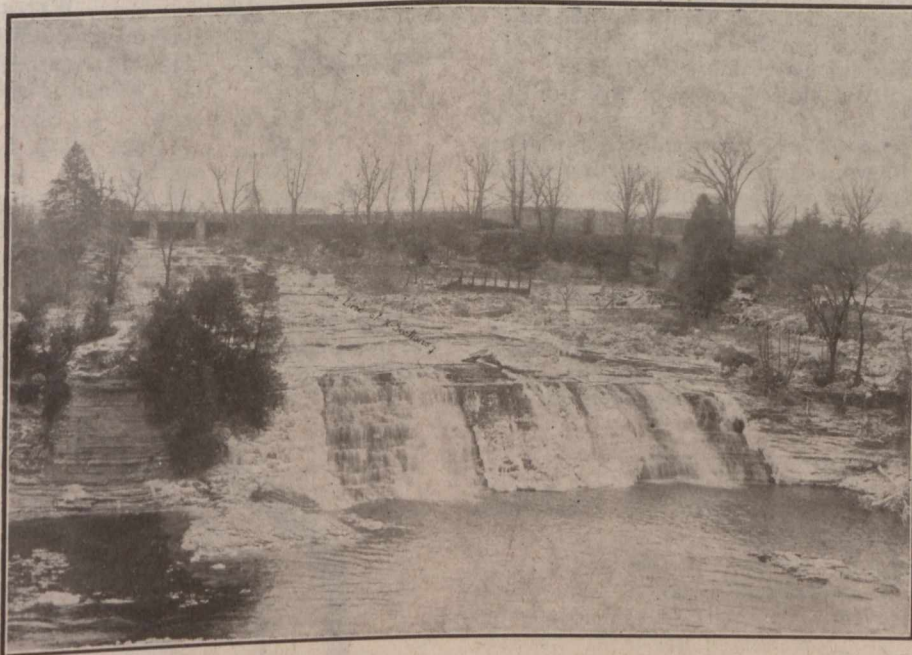
SITE OF RANNEY'S FALLS DEVELOPMENT, LOOKING FROM LOWER END OF TAILRACE TOWARD INTAKE SLUICEWAY IN BACKGROUND
