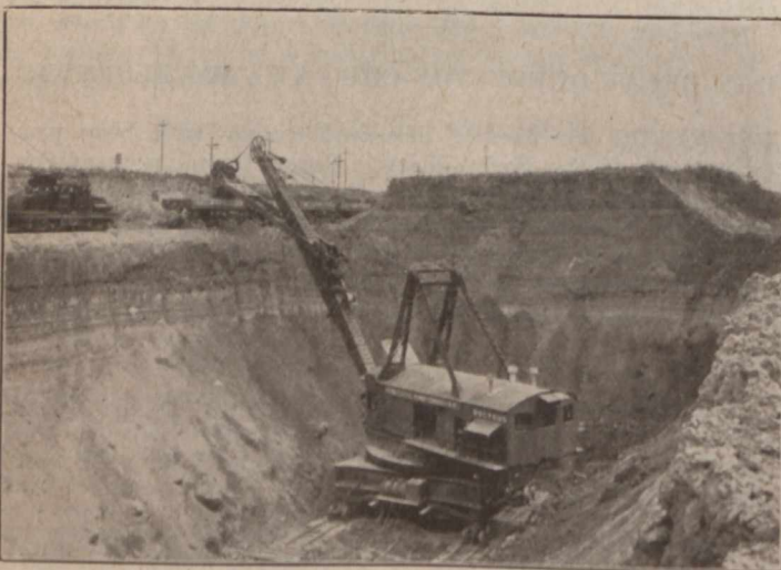
FIG. 1—BUCYRUS SHOVEL WORKING AGAINST 90-FT. CLIFF DURING POWER-CONSUMPTION TEST
