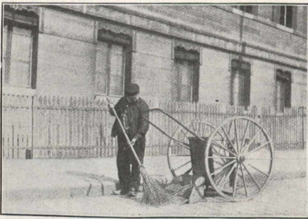
Fig. 3—Iron Wheelbarrow for Removing Sweepings.
