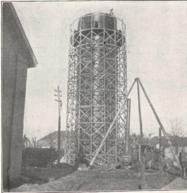
Stand Pipe 20 Feet, Diameter 100 Feet High During Erection
