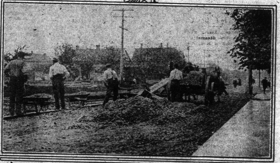
DUMPING THE CRUSHED ROCK
