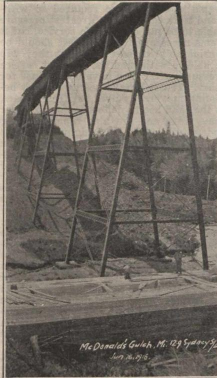
McDonald's Gulch, showing construction of rail concrete culvert, before filling commenced.
