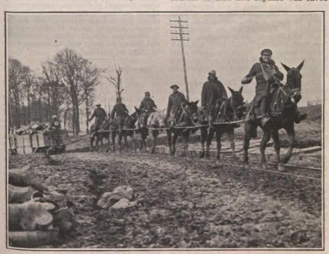
A mule tram drawing ammunition, on a light railway, behind the Canadian lines at Vimy Ridge.
