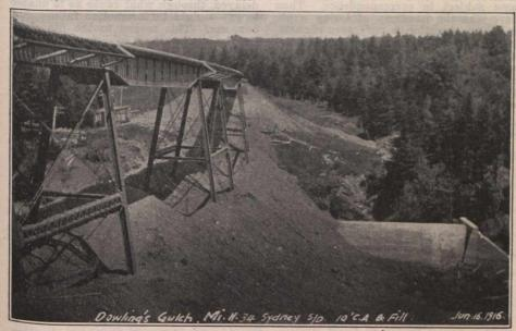
Dowling's Gulch Steel Viaduct, showing culvert and filling.
