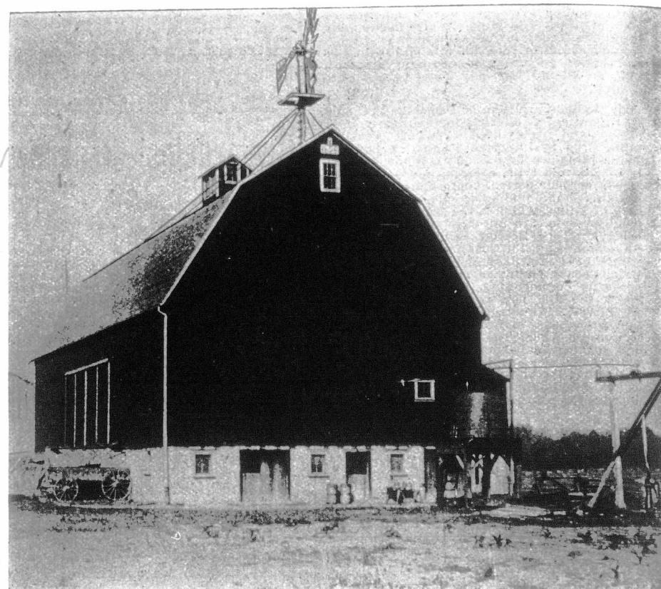
Stock barn of Mr. John D. Ferguson, in the township of Yarmouth. Dimensions of the building, 80 x 48 feet; foundations of concrete, 2 1/2 feet deep. Floors and roof, cellar all of Thorold Cement.
