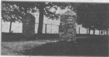
This massive colunna are simply constructed of ordinary boards capped with cement. Entrance to the garden home of Albert Jull, Bran. Co., Ont. —Photo by an editor of Farm and Dairy.
