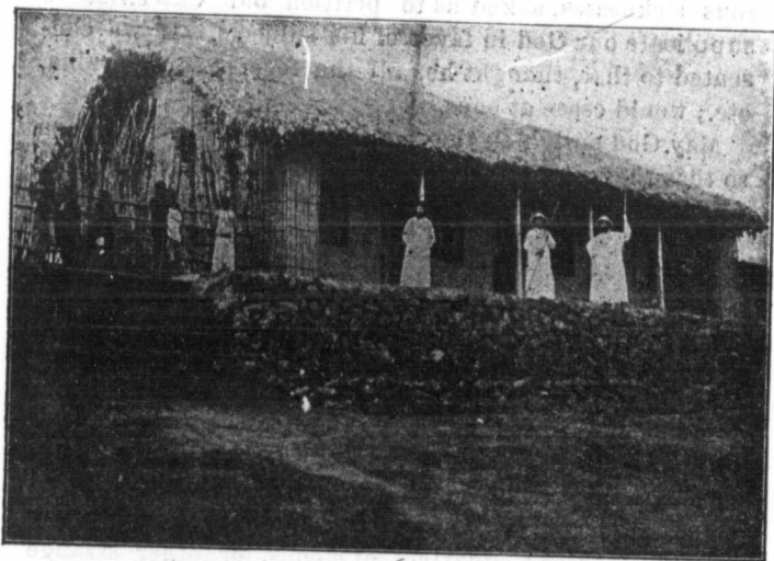
Our first installation.
