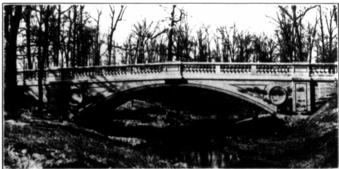
Fig. 26—Franklin Bridge, Forest Park, St. Louis, Mo.
