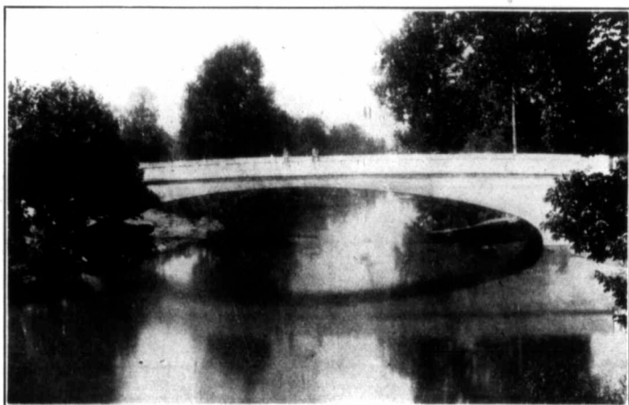
Fig. 25—Bridge at Yorktown, Ind.
