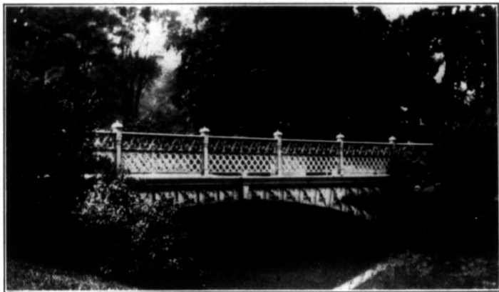
Fig. 7—Bridge in Belle Isle Park, Detroit.
