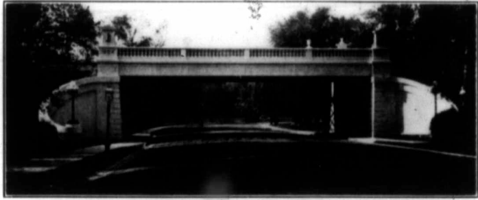
Fig. 2—Railroad Bridge at Entrance to Forest Park, St. Louis, Mo.
