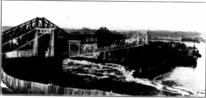
Fig. 14—Bridges at St. John, N.B.
