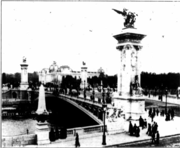
Fig. 3—Alexander III. Bridge, Paris.
