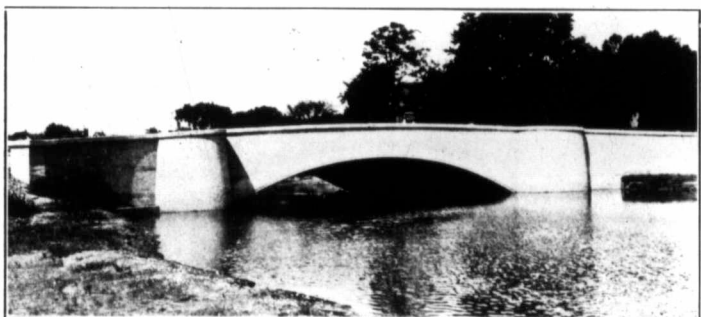
Fig. 27—Auburn Street Bridge, Medford, Mass.
