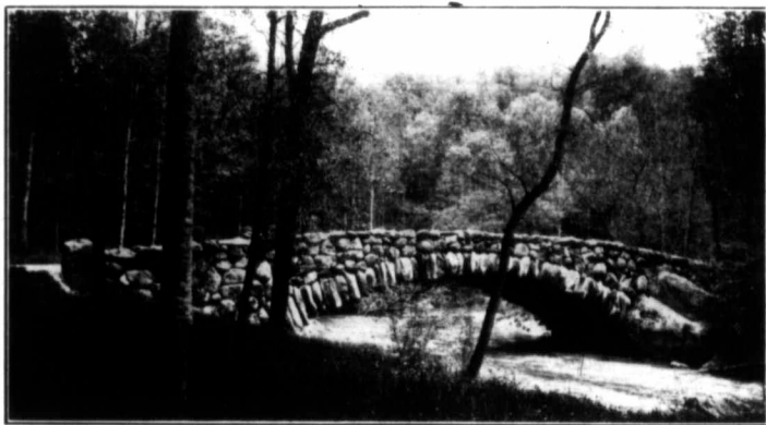
Fig. 5—Bridge in National Park, Washington, D.C.
