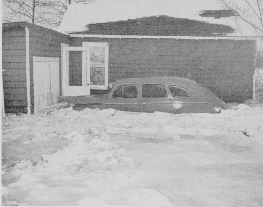
Bowness flood damage.
