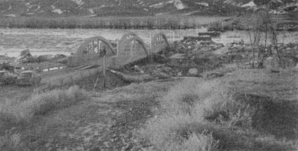
Above —Bridge from north shore shortly after its collapse.
