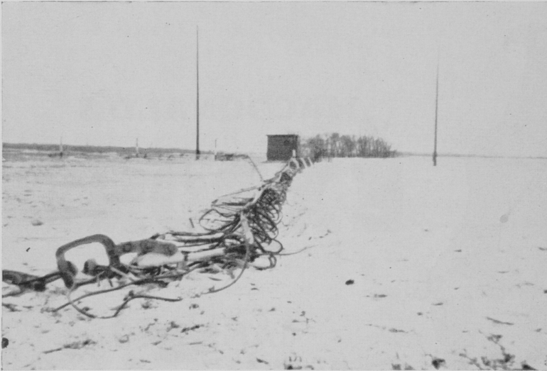
The wreck of the tower. Bodies of two of the workers were found in the flattened portion in foreground.
