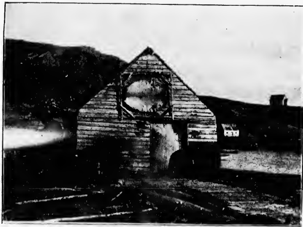
FIG. 7.—Storehouse at Cape Charles Harbour, with a seal skin stretched out to dry. Chapel on the hill.
