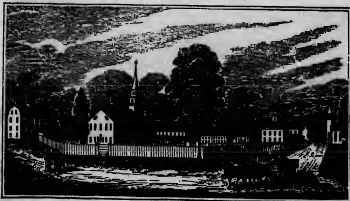
Western view of the public buildings at Goshen.
