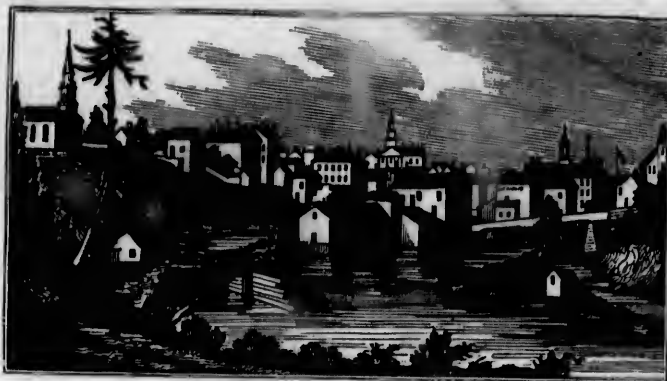
East view of Seneca Falls village.
