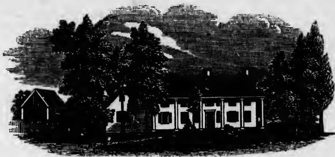
Schuyler mansion-house, Schuylerville.
