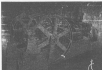
Westinghouse Induction Motor Driving Aldrick Pump.
