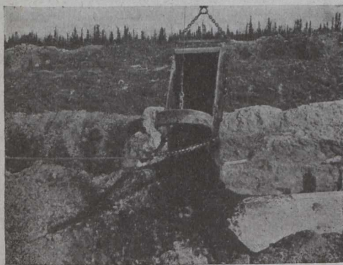
Backfilling.—Second Operation. Depositing muskeg on top of the sandy clay.
