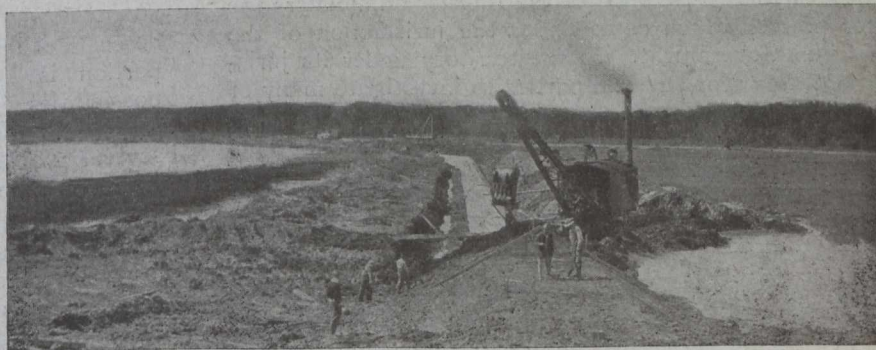
Backfilling at Indianhead Bay.
