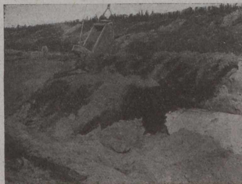
Backfilling.—Third Operation. Placing sandy clay on top of the muskeg.
