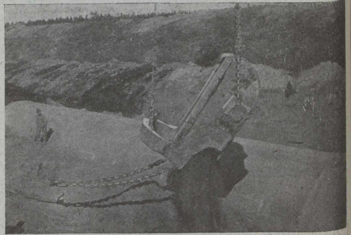
Backfilling.—First Operation. Depositing sandy clay alongside the aqueduct.
