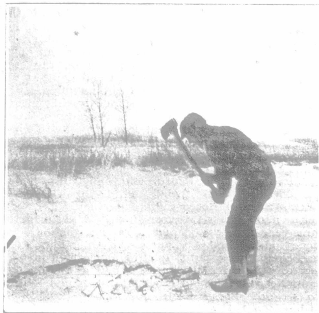
Digging for Water.
