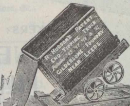
1—R. H.'s Patent Steel End Tip Wagon
