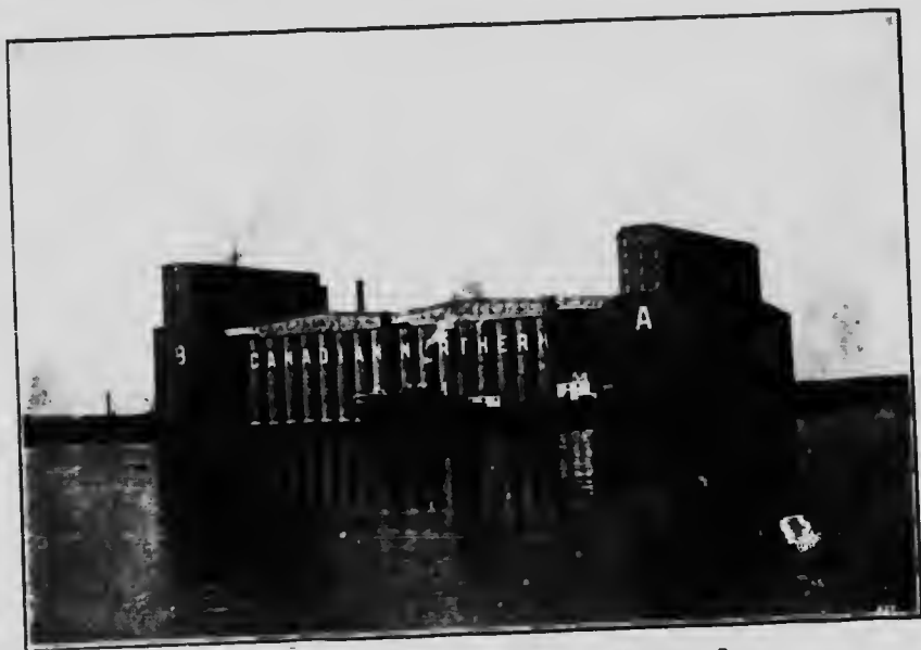
Canadian Northern Elevator, Port Arthur, Ont. Largest Elevator in the World. Cap., 7,250,000 bu.
