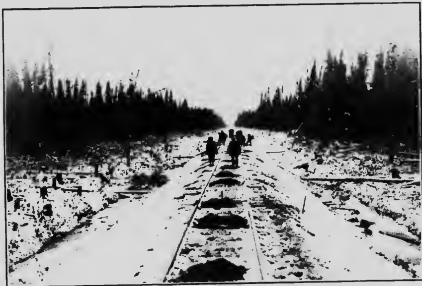
Railway Construction Scene in Northern Ontario
