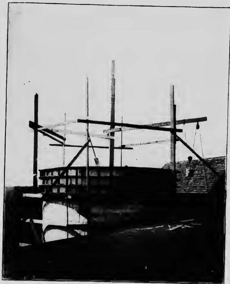
(Fig. 5.) Showing method of erecting staging.
