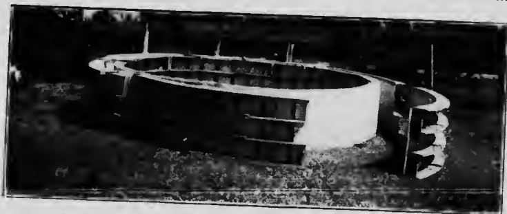
(Fig. 4.) Forms detached from first course above foundation.
