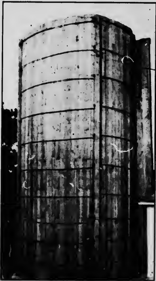
(Fig. 19.) Stave Silo with posts instead of lugs.
