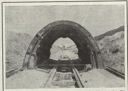
Winnipeg Water will come for 100 miles through an aqueduct of which this is a section. is the new underground riverway that will provide future greater Winnipeg with a maximum of 88,000,000 gallons a day. The aqueduct railway runs along the bank to the right.
