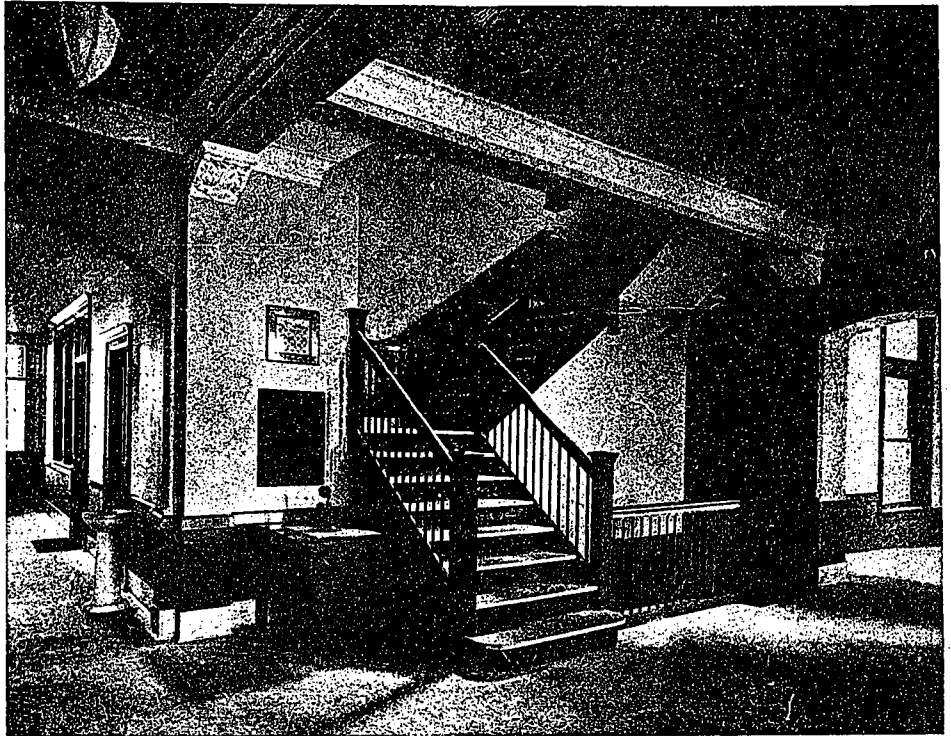
CORRIDORS AND STAIRS. STEEL COMPANY OF CANADA'S OFFICE BUILDING, HAMILTON, ONT.
