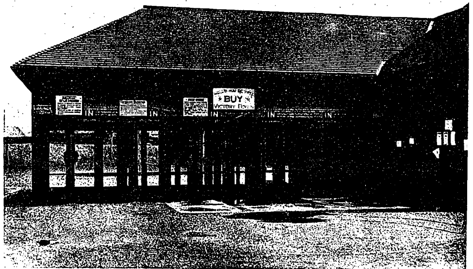
ENTRANCE TO PLANT, STEEL COMPANY OF CANADA.
