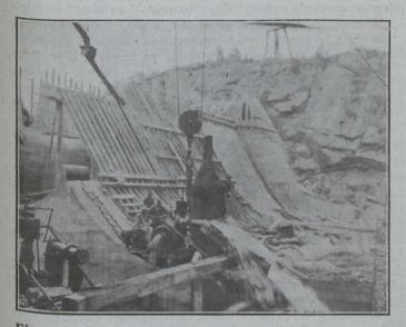
Fig. 4.—Pumping Out Sluice Pipe Chamber Preparatory to Connecting Sluice Pipe with Sluice Valves
