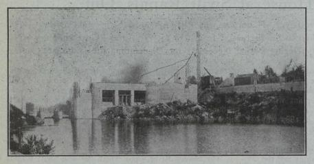
Fig. 2.—View Taken Looking Downstream, Showing Wheel-pit House, Entrance to Canal and Dam Partly Built
