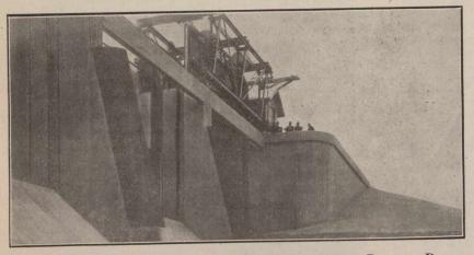
Fig. 2.-Massive Abutment and Pier Construction, Bassano Dam.
