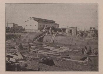
Fig. 4.—Placing of Column Footings, Transformer Station.
