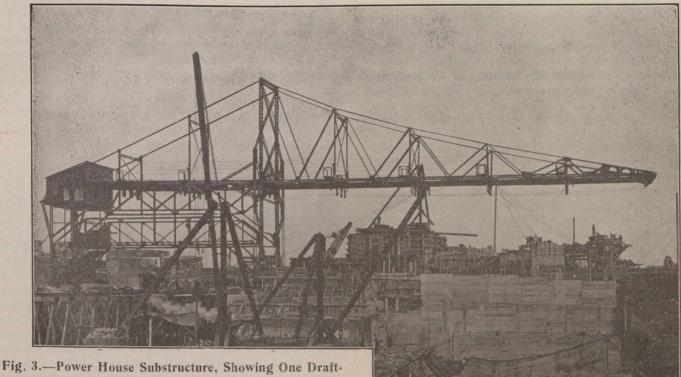
Fig. 3.—Power House Substructure, Showing One Draft-Tube Under Construction.
