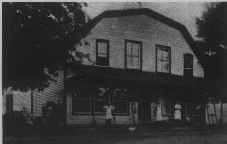
Fawthrop Bros., Cornwall—the present building. A. Fawthrop is standing to the left of the door.
