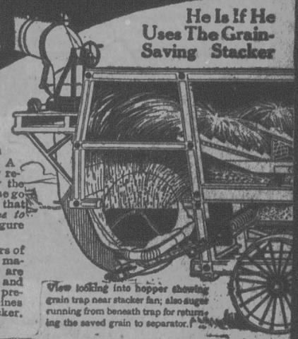
View looking into hopper showing grain trap near stacker fan; also auger running from beneath trap for returning the saved grain to separator.
