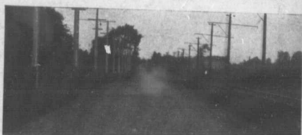
Gull-Prison Macadamized Road, Waterloo Co., Ont. Treated with "Tarvia B." 1914
