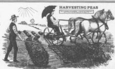
The Genuine Tolton Pea Harvester with new Patent Side-delivery Self-buncher at work
