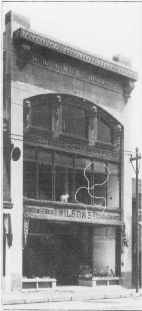
Store for THE HAROLD A. WILSON CO., LIMITED, TORONTO. Chapman & McGiffin, Architects.
