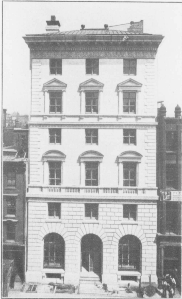
THE ROYAL BANK OF CANADA, TORONTO. Carrère & Hastings } Associated Architects. Eustace G. Bird }
