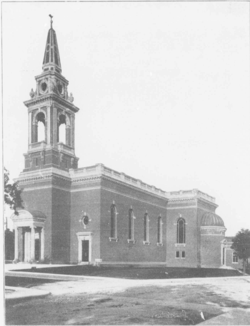
CENTRAL PRESBYTERIAN CHURCH, HAMILTON, John M. Lyle, Architect.
