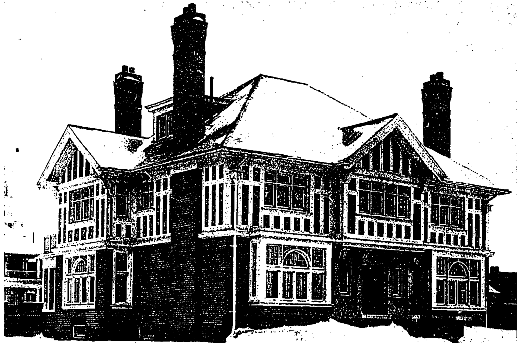
Residence of N. Hillary, cor. Bernard Ave. and Admiral Road, Toronto. F. S. Baker, F.R.I.B.A., Architect.
