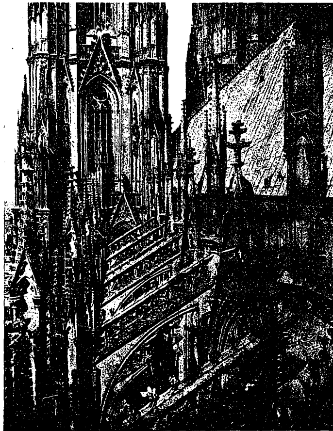
Flying Buttresses of the Cologne Cathedral.
